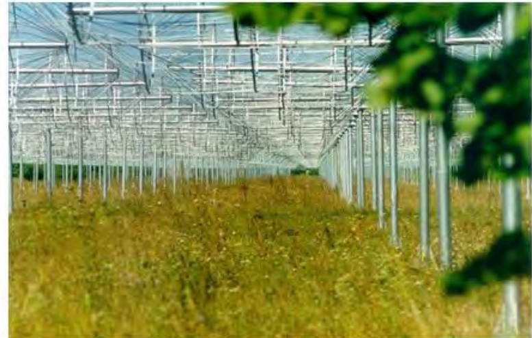
Fig.1. The UTR-2 radio telescope, N-S arm (1.8 km×60m) f = 8...32 MHz, A_{\text{eff max}} = 150\,000 sq.m
