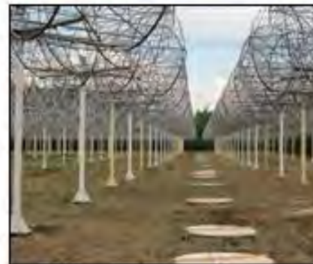
Fig.2. URAN-1...URAN-4 radio telescopes, (angular resolution is near one arcsec for the base line 950 km )
